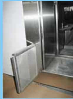
Heater battery filter with easy access
